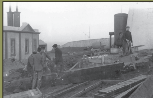
Radar station under construction in 1939. (courtesy collection of Lt Dunworth via Squadron Leader Mike Dean, MBE)
