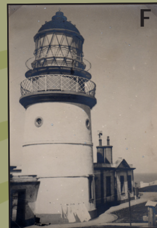
During wartime, soot and brown clay were added to the limewash coating the lighthouse tower to help it blend into its surroundings.
