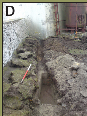
A buried brick-built tank was found next to the foghorn during restoration works. This may have been the storage pit for the Lewis gun ammunition.
