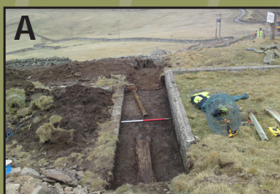
Foundations of the barrack blocks which housed the army guard for the radar station.
