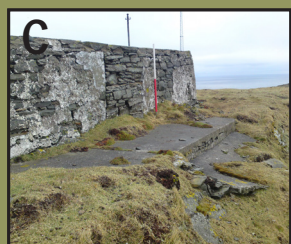
This concrete platform and blocked up entrance within the stone wall may be a defensive Lewis gun platform.
