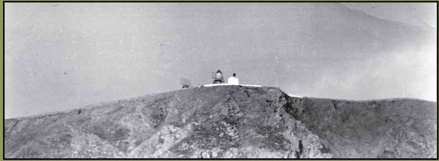
Sumburgh Head Radar Station as viewed from aboard the Good Shepherd at sea
